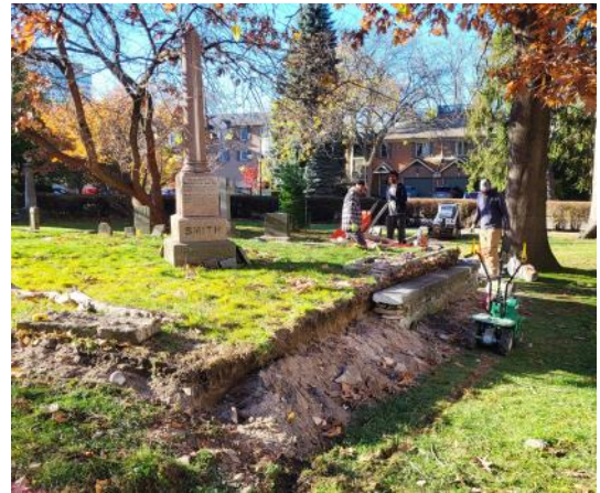
Cemetery Retaining Wall Repair
